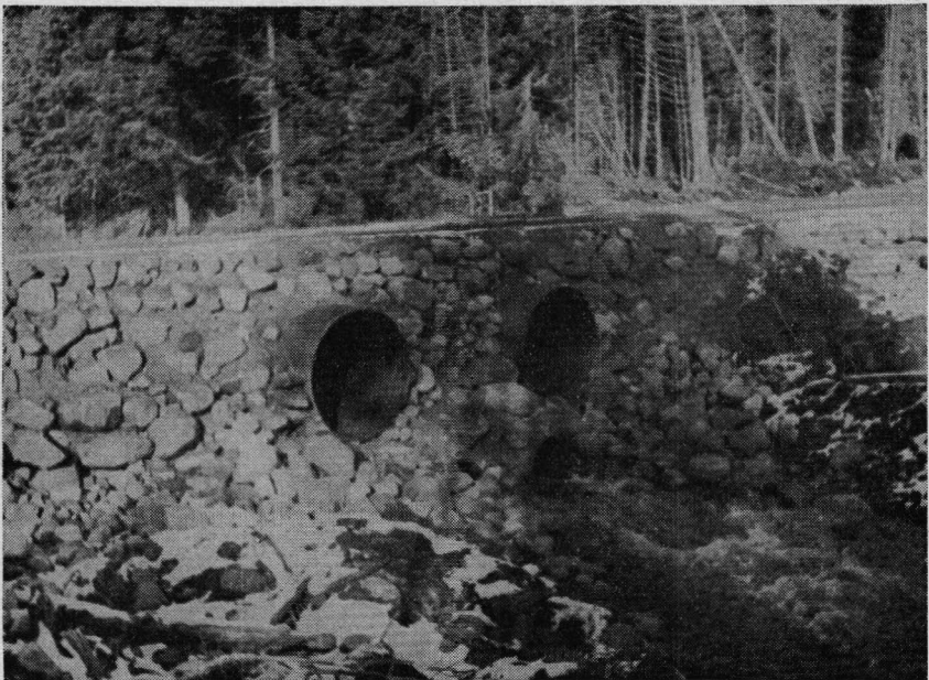
Figure 4. Moose Pond Dam showing two 5-foot pipes for flood spillways.
