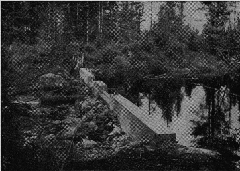
Figure 2. Sperry Pond Dam.
