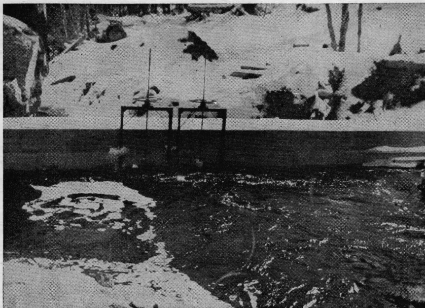
Figure 3. Round Lake Dam—Lake Surface above two 36-inch valves.
